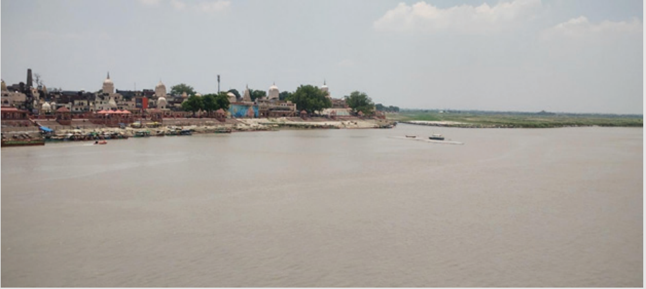
Fig. 4 View of the Ayodhya riverfront, engineered ghats and temple on the stable right bank, contrasted with the open floodplain of the opposite bank, Saryu River.
