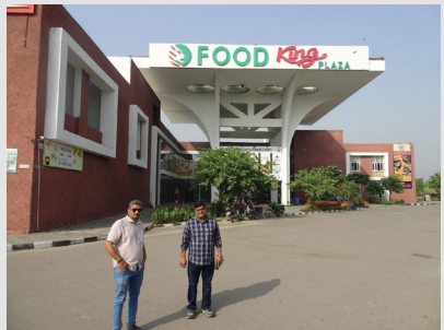
View during inspection for food facility located in the Lucknow-Agra expressway
